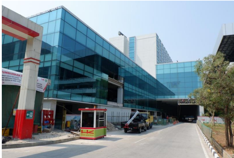
Gambar 2. 1 Tampak Samping Proyek Airport Hotel International Terminal 3 Ultimate
