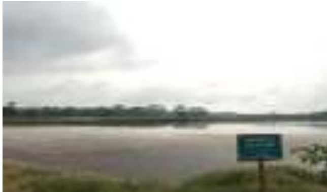
Gambar 2.6. Kolam An aerobik 2
