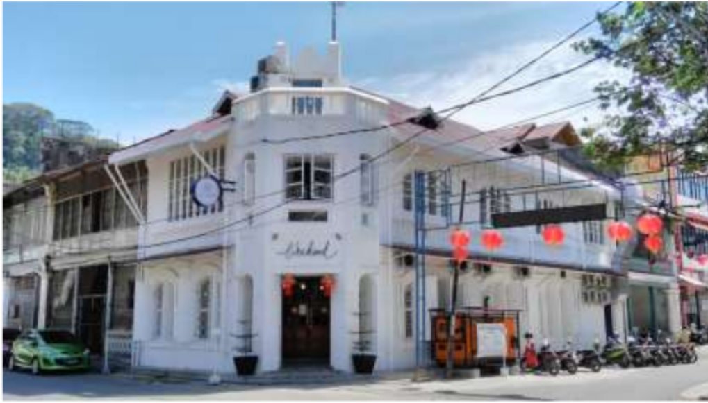
Gambar 5- 25 Bangunan Weekend Cafe
