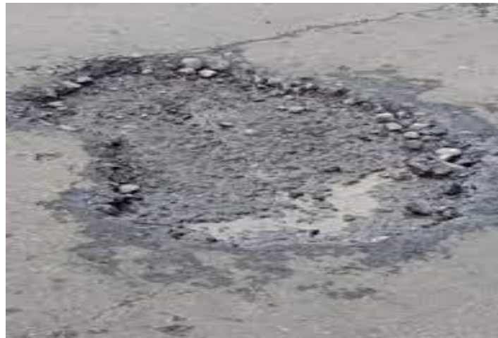
Gambar 2.18 Pelapukan dan Butiran Lepas ( Weathering and Raveling )
