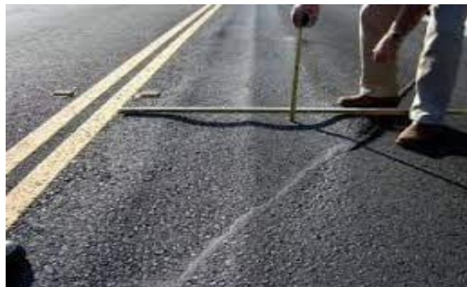
Gambar 2.4 Alur ( Rutting )
