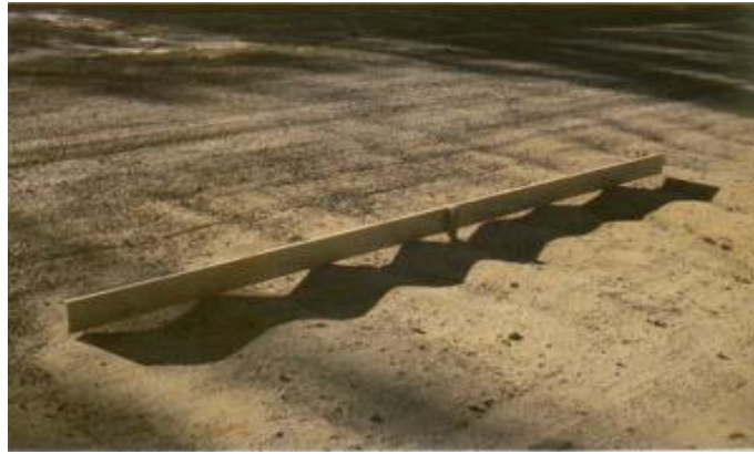
Gambar 2.3 Bergelombang ( Corrugation )
