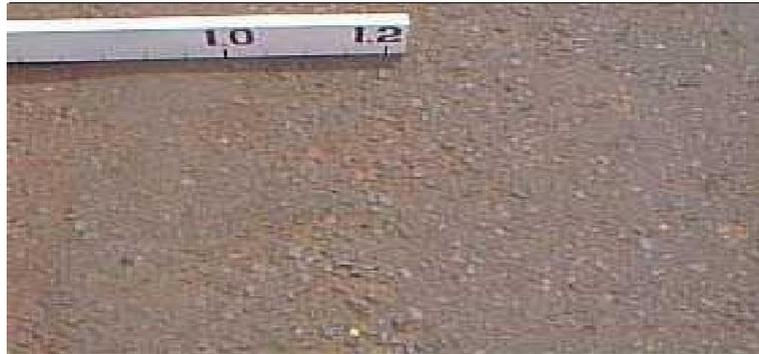
**Gambar 2.15 Agregat Licin (*Polished Aggregate*)**
