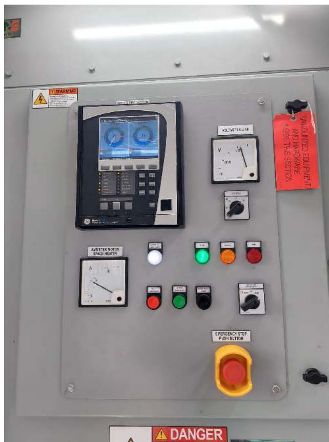
Lampiran. 7 Gambar MCC pompa WIP petani GSPanel MCC pompa WIP Petani GS
