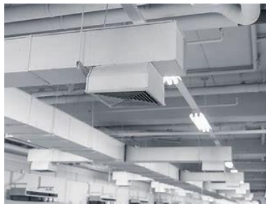
Gambar 2. 10 AC Ceiling Mounted Ducting
