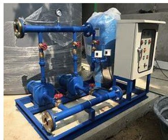
Gambar 2. 47 Booster Pump
