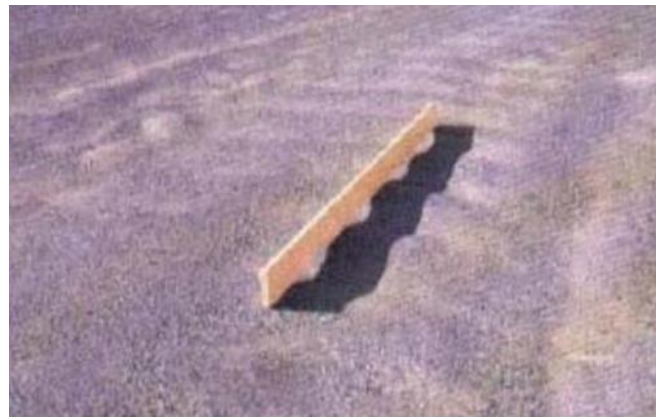
gambar 2. 7 Contoh Kerusakan Keriting ( Corrugation ) (Sumber : Bina Marga no.03/MN/B/1983)
