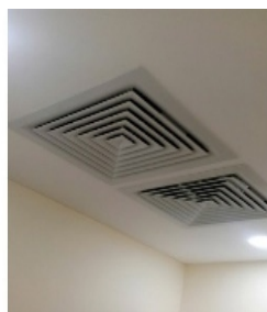
Gambar 3.28 Diffuser
