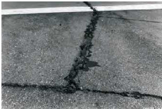
Gambar 2.13 High Severity
