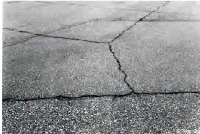
Gambar 2.11 Low Severity
