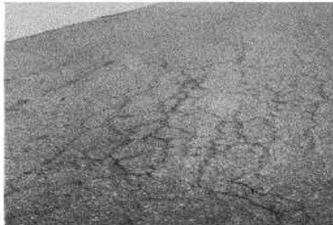
Gambar 2.2 Medium Severity
