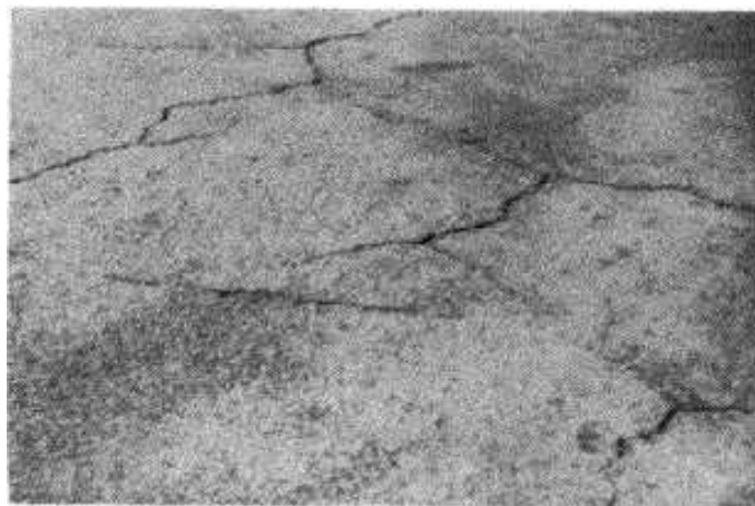
Gambar 2.5 Low Severity
