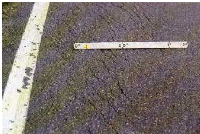
Gambar 2.22 Slippage Cracking
