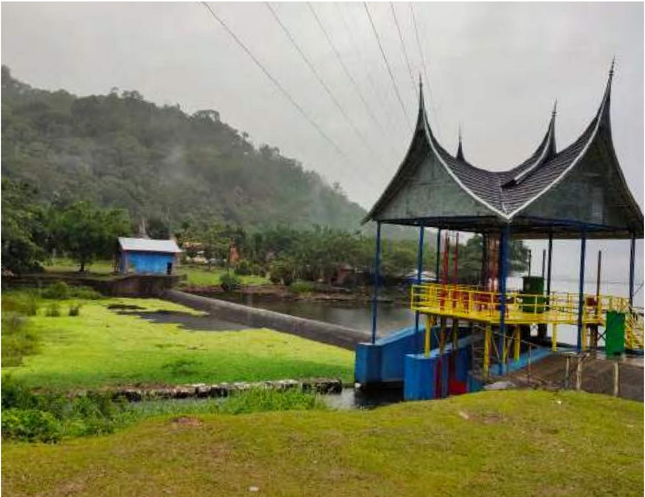
Dam Weir PLTA Maninjau 2019
