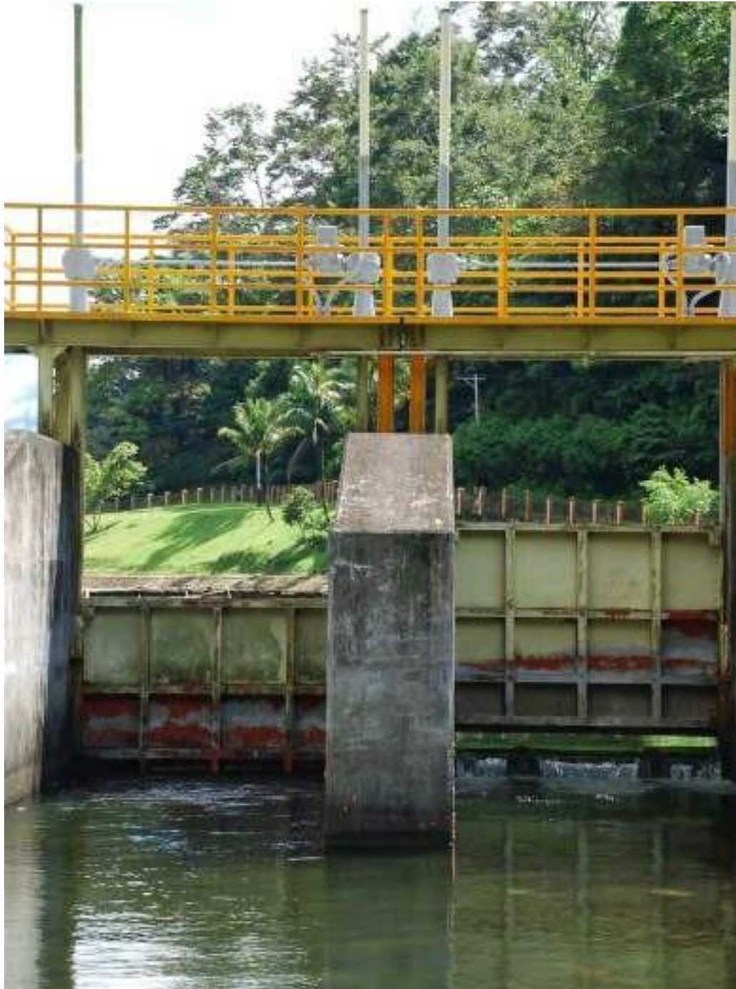
Dam Weir PLTA Maninjau 2013
