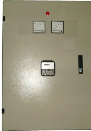
Gambar 3.8 Unit Panel Distribusi PLTS Terpusat.
