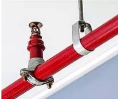
Gambar 2.11 Sprinkler Upright
